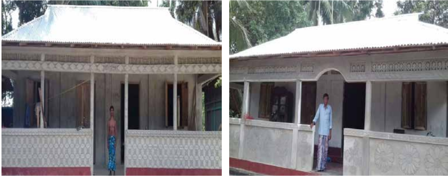
Houses constructed under BLC component of PMAY(U) using new technology in Melaghar, Tripura
